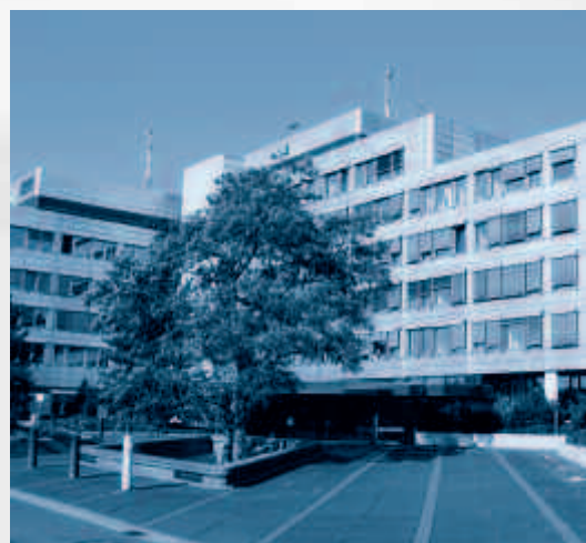
Photos: Views of the BKA in Wiesbaden (above), Berlin (centre) and Meckenheim by Bonn (below)
