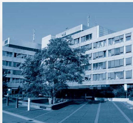
Photos: Views of the BKA in Wiesbaden (above), Berlin (centre) and Meckenheim by Bonn (below)
